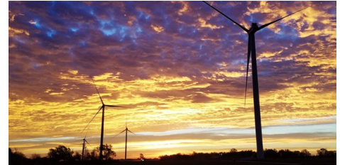
EDF's Great Western Wind Project in Oklahoma | EDF
