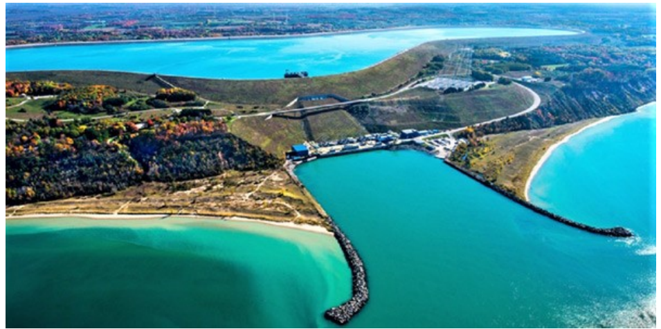
Ludington pumped storage facility | Consumers Energy
